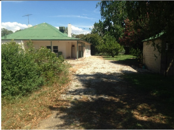
Plate 10: House and out-buildings on the terrace. Assumption is that these areas are disturbed.
