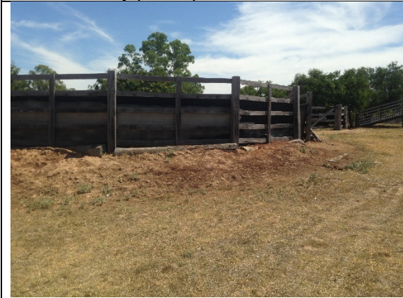
Plate 9: Infrastructure development on the terrace.
