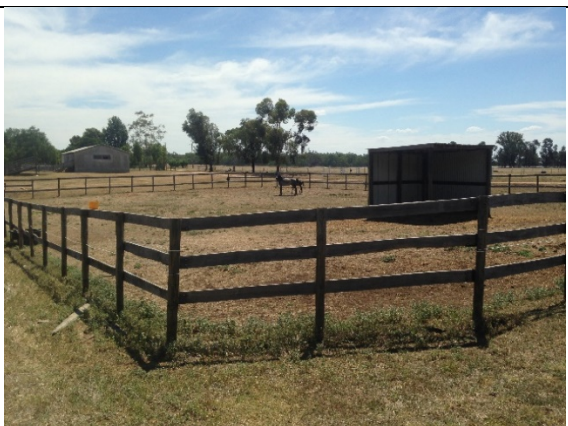
Plate 8: Infrastructure development on the terrace.
